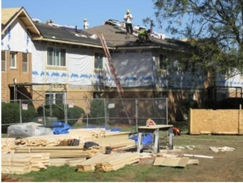
Photo by STAN BULLARD Taking the mansards out of mansard roofs on a North Olmsted apartment complex was no small undertaking.
